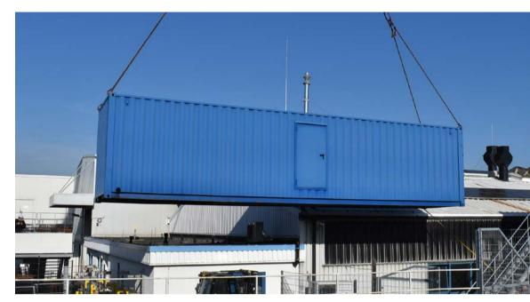
Installation of the biofilter in container form.
